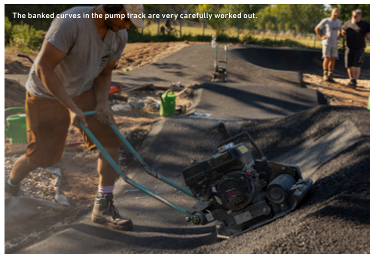
For working on the curve, the Schneestern employees have adapted the APF 10/33 vibratory plate from Ammann. The drawbar was moved.
