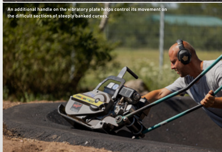
The plate was ground into a convex shape. This allows perfect modelling of curves.
