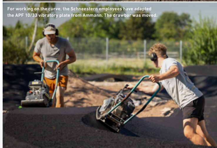
An additional handle on the vibratory plate helps control its movement on the difficult sections of steeply banked curves.
