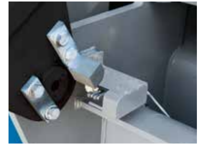
Secondary boom hoist limiting device that cannot be released by the operator
